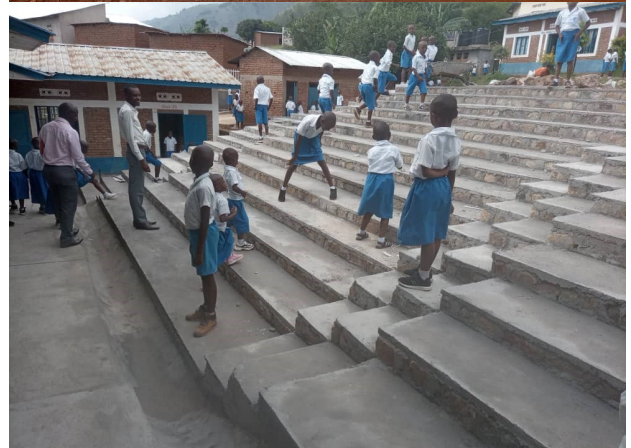
Top: New playground provided by Sterling Dr. Church of Christ. Bottom: New steps for Mango Tree School.
