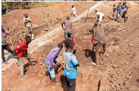
Top: old road continues to wash away. Bottom: Great progress on new road!
