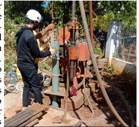
Drilling new well in leper village.
