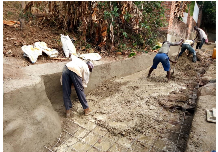
Phase One of the drainage system is nearly complete.
