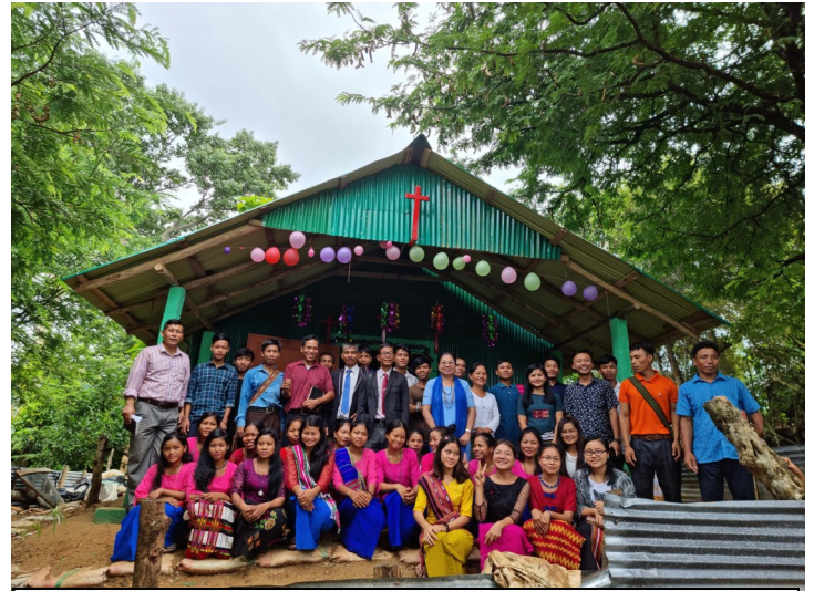
They are so proud of their new church building and thank God for the Global Outreach donor who provided the roof.
