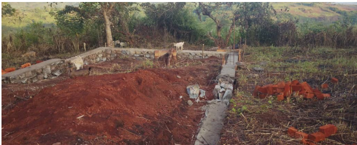
Foundation of the new girls home needed lots of large rocks.
