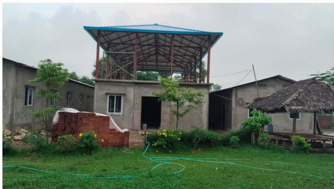
This picture shows the boys and girls dormitories with the new multipurpose building under construction. The thatch roof structure on the right is the current dining room.
