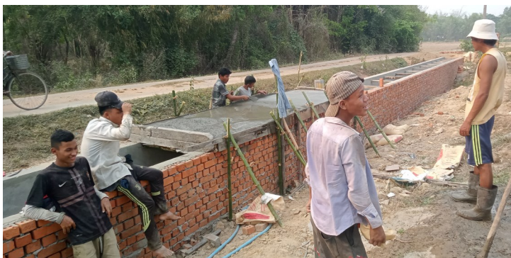
One hundred-thirty foot drainage ditch has been completed.
