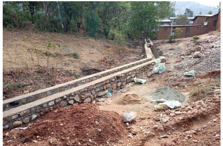
Trenches such as these will provide better drainage to avoid future flood damage.
