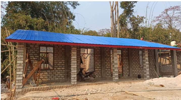
By February 2023 construction of the women's dormitory was well under way.
